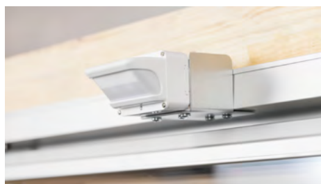
Anti-sweat Sensors & LED Motion Sensor Installed
