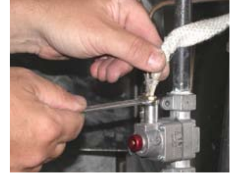
12. Thread the thermocouple fitting into the body by hand. When you can no longer tighten by hand, use a 3/8" wrench to make snug. A good rule is giving a 1/8 turn after finger tightening. DO NOT OVERTIGHTEN as it will damage the control. Turn on gas, check for leaks, and relight pilot.
