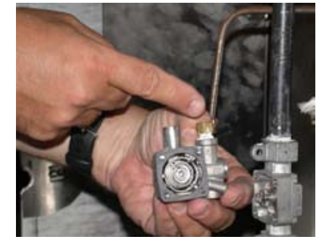
6. Remove brass adaptor attached to the safety head and install on the new head.
