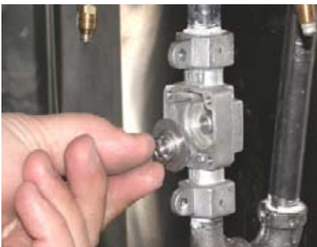
7. Remove and replace the spring/magnet assembly.
