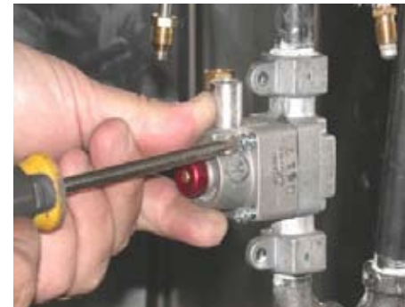
4. Remove the screws from the safety head.
