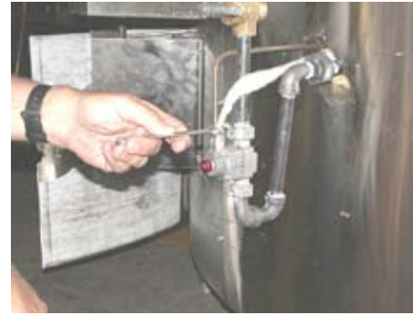
2. Using a \frac{3}{8} " wrench, remove the brass thermocouple fitting from the safety control.
