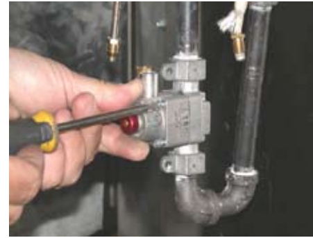
10. Mount the safety head and replace the screws.
