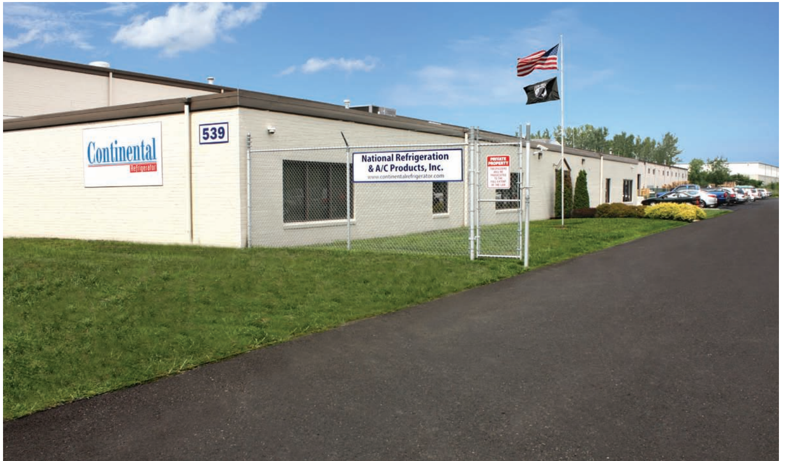
Bensalem, Pennsylvania Continental Refrigerator, Dunksferry Facility
