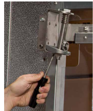
Hinge cam block adjusts with phillips head screwdriver.
