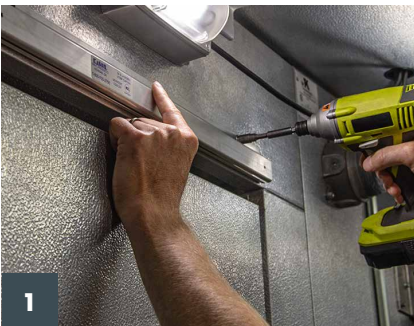
1 Attach mounting bar
