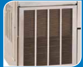
Easy to access mechanical sections
