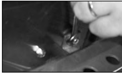
Removing the bracket nut
