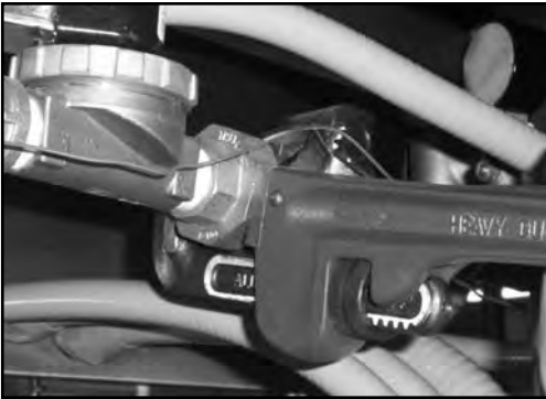
Loosening the union on the incoming plumbing
