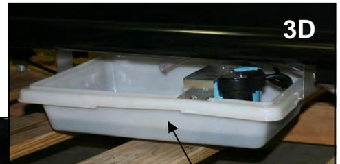
View of Condensate Pump Pan (Positioned Properly and Fully Connected)
