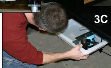
Sliding Condensate Pump Pan under case
