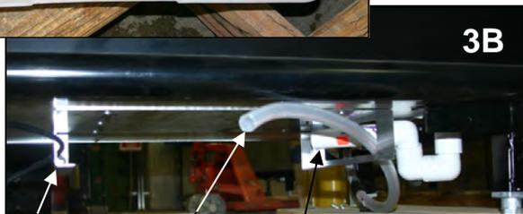
Condensate Pump Pan Support Bracket (one at either side)
