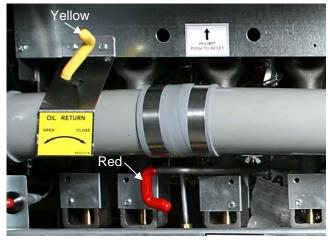
The red handle is attached to the drain valve. The vellow handle is attached to the oil return valve.
