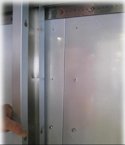
Remove the pilaster strips from the back wall. So the rear pilaster support can be installed. Eight (8) of these screws will be replaced when the pilaster are removed.
