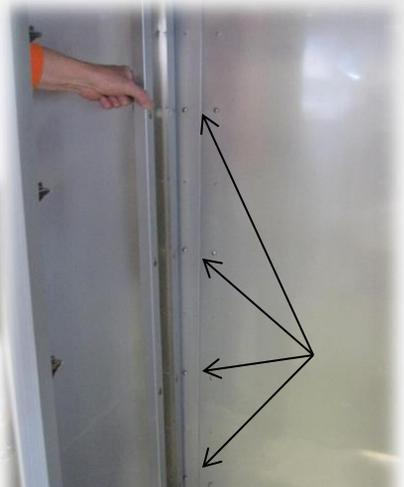
Install (8) of the screws removed in the last step in the 3rd, 5th, 7th & 9th set of holes in the back liner. (Counting down from the top.) The screw head should be 1/8" from the back wall to allow the Rear Pilaster Support to be slid over the keyhole slot.
