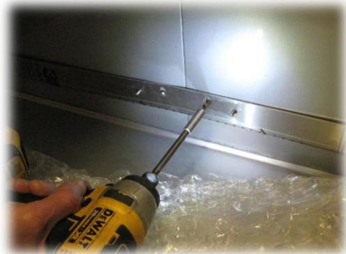
Install the "Bottom Rear Bracket" using the bottom holes for the center pilasters (Above). Install the supplied 3/4" long screws into the bottom holes of the Side Brackets to hold the ends of the Bottom Bracket. (Do not tighten these screws at this time. These screws will be tightened after the Back Spacer is installed.)
