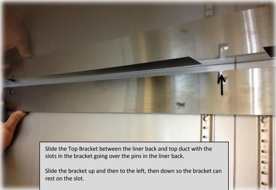
Slide the Top Bracket between the liner back and top duct with the slots in the bracket going over the pins in the liner back.
